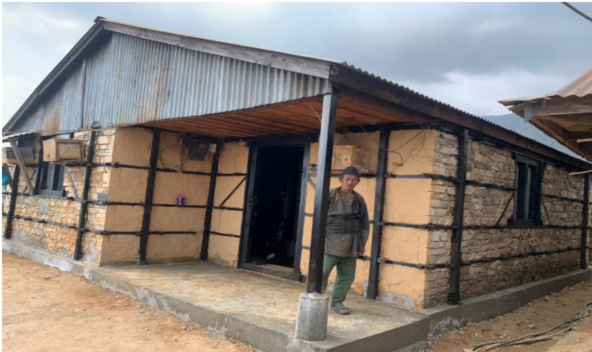
A house after completed restoration works at Helambu-5.
